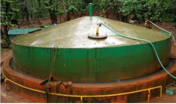
BIO GAS DIGESTOR
