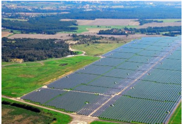
Waldpolenz Germany- Solar plant- 40 MW
