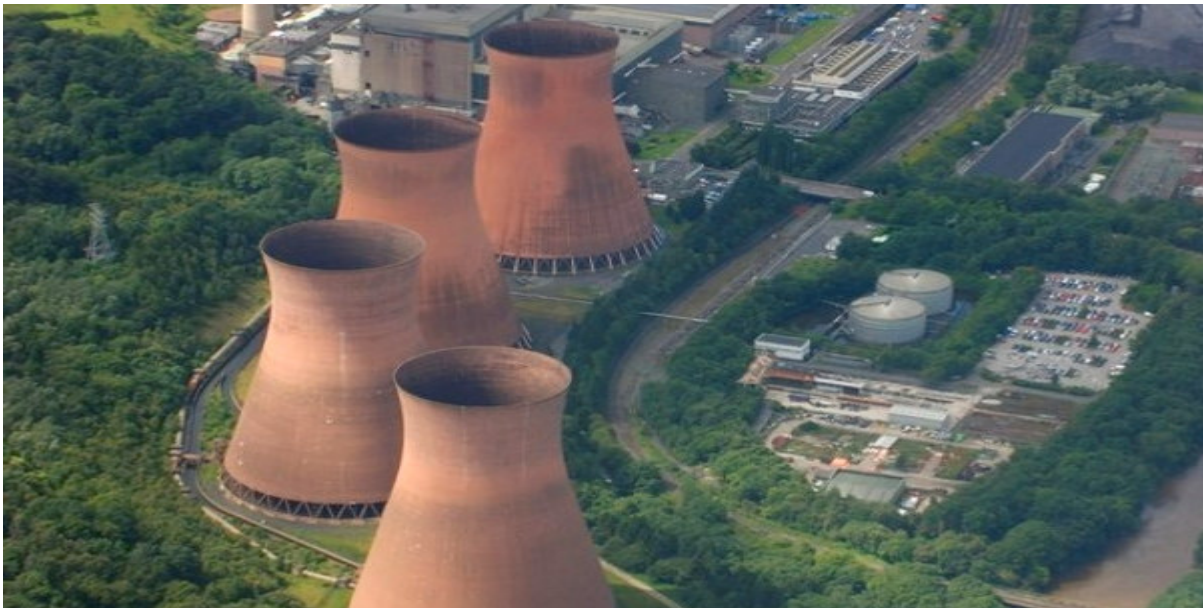
BIO GAS POWER PLANT UK--740 MW
