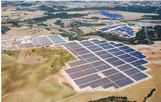
Solar power plant-Spain-60 MW
