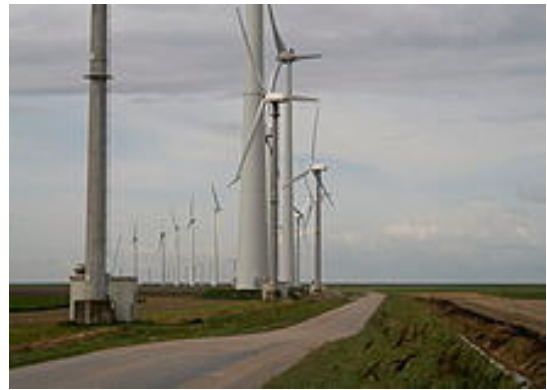
Westereems wind farm Netherland-156 MW
