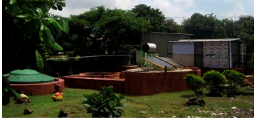
TYPICAL BIO GAS PLANT FOR HOME
