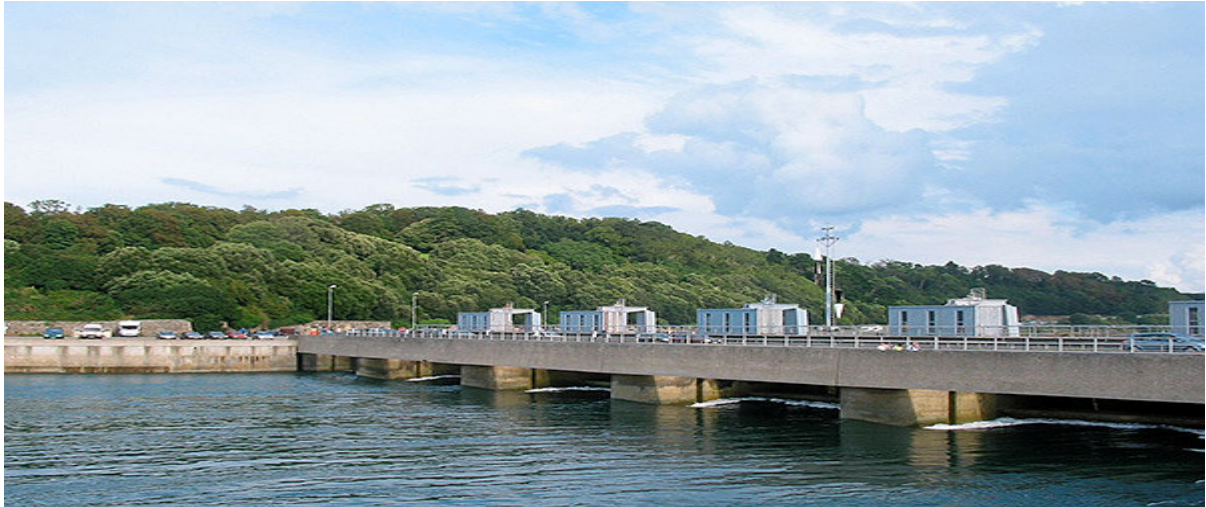
La Rance Tidal Power Plant, France - 240MW
