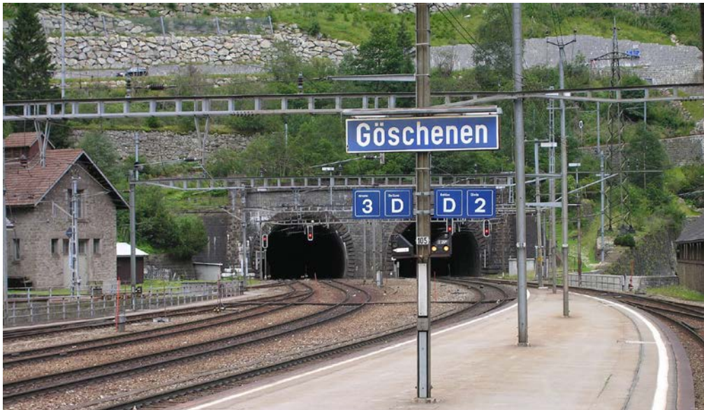
Figure 6: Northern end of the Gotthard railway tunnel, Göschenen, Switzerland
