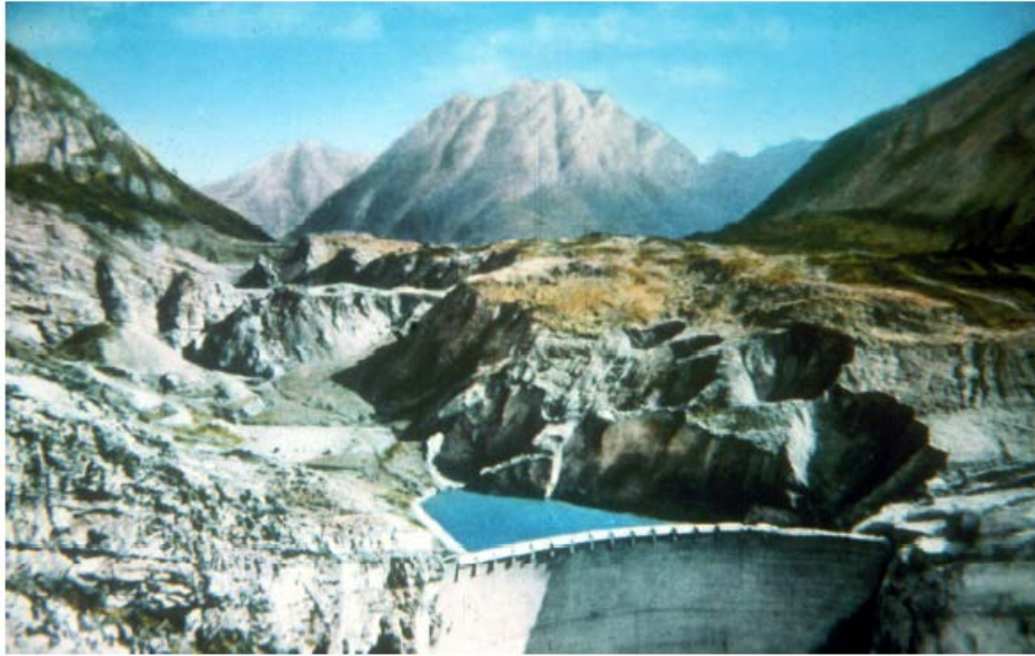
Figure 8: Vajont dam, Longarone , Italy
