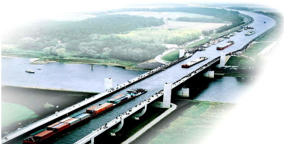
Figure 1. Canal crossing a natural drainage
