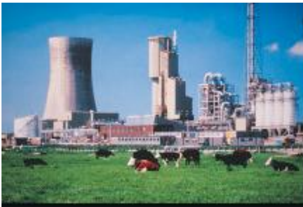
SCP Processing Plant
