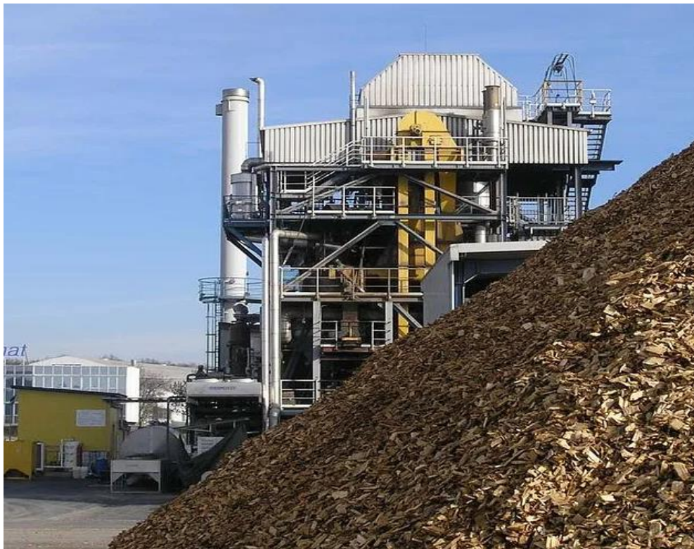
Views of Typical Biomass Gasification (Power) Plant (Source:BioEnergy Consult, July 2019)
