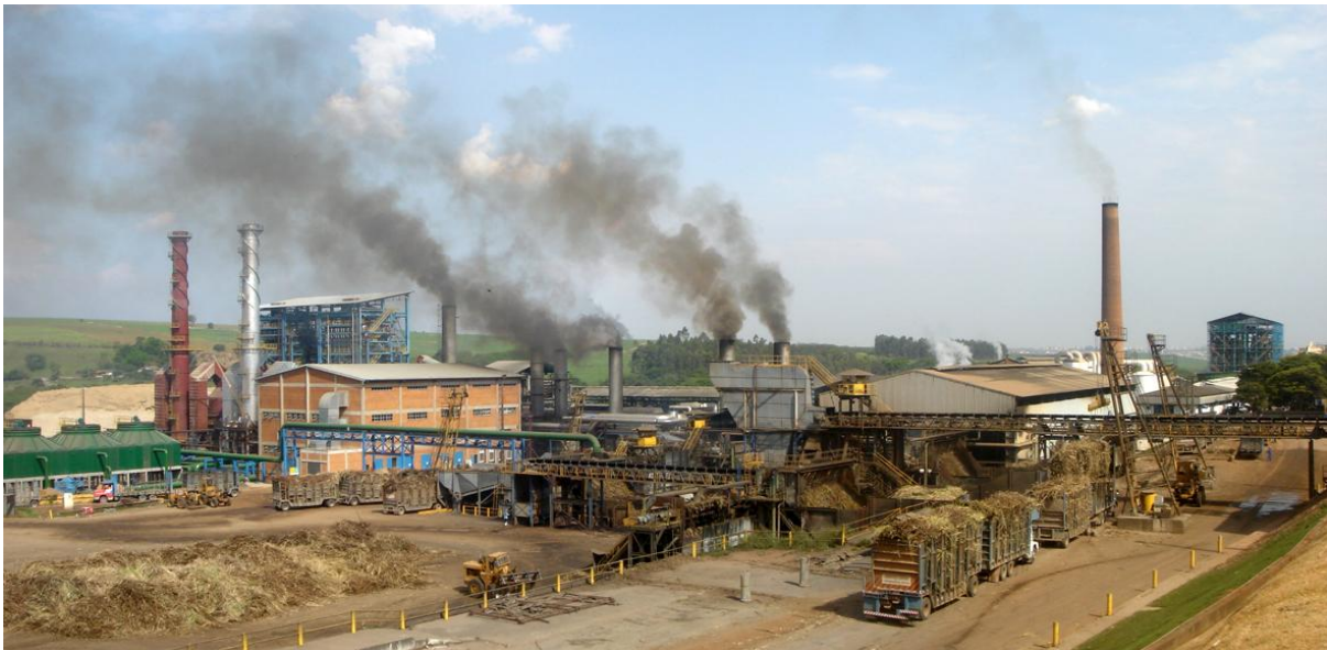
Sugarcane Ethanol Plant in Brazil
