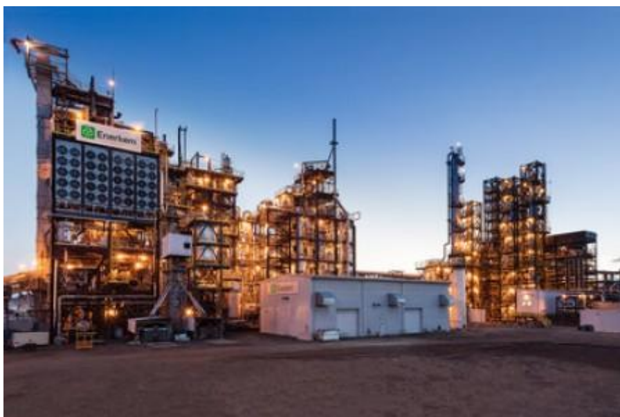
Figure-29: A picture of Enerkem's state-of-the-art Edmonton (Canada) biofuels facility, the world's first commercial scale plant to produce cellulosic ethanol made from non-recyclable, non-compostable mixed municipal solid waste. (CNW Group/Enerkem Inc. 2017)
